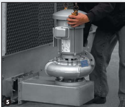
5 Mount Pump and Piping
