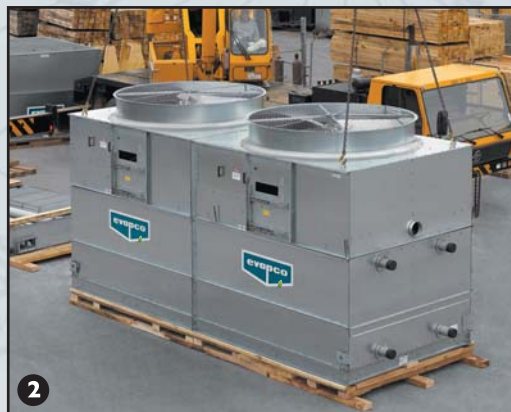
2 Mount Fan Section to Coil Section
