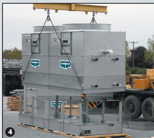
4 Mount Coil/Fan to basin Section
