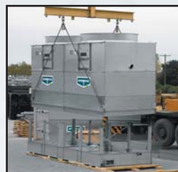
Mount Fill/Fan to Basin Section
