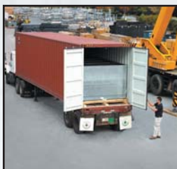
Unload Unit from Container
